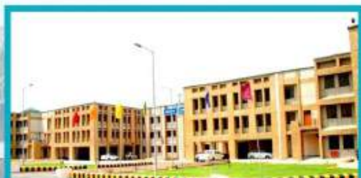
ADMINISTRATIVE BUILDING SVPUA&T, MEERUT
