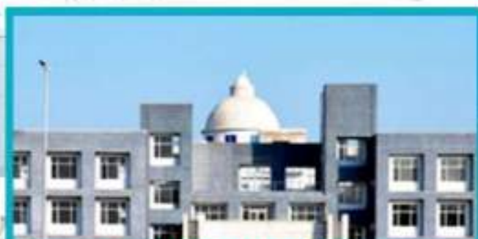
ADMINISTRATIVE BUILDING BUA&T, BANDA
