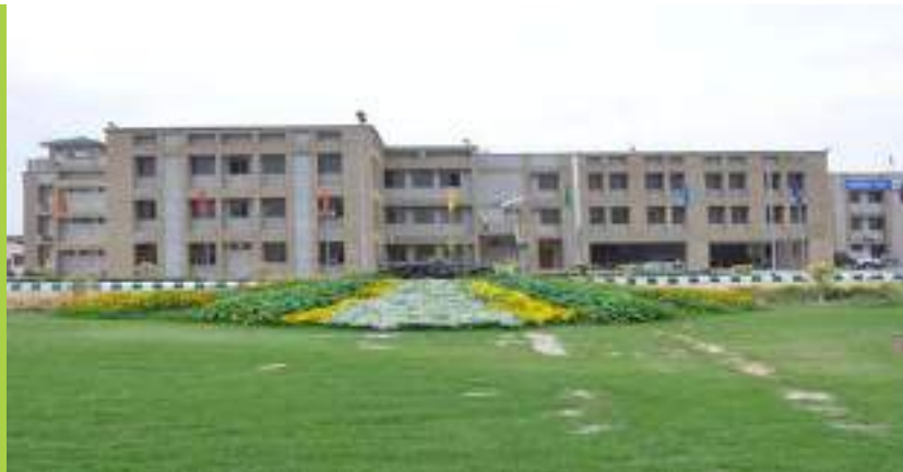
Administrative Building SJUA&T, MEERUT
