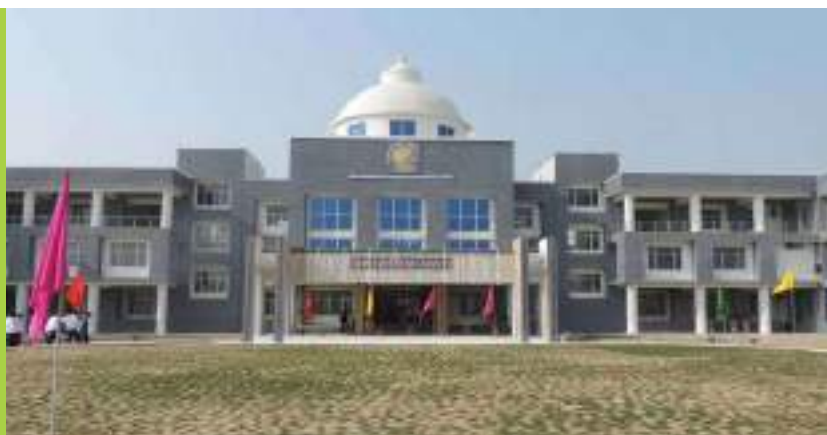
Administrative Building BUAT, BANDA
