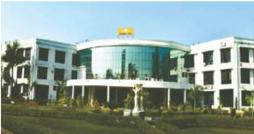
Administrative Building ANDUA&T, AYODHYA
