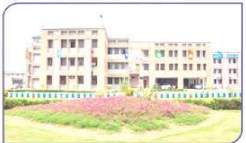
ADMINISTRATIVE BUILDING SVP&T, MEERUT
