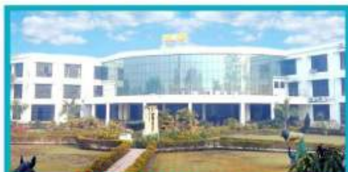
ADMINISTRATIVE BUILDING NDUA&T, KUMARGANJ, AYODHYA
