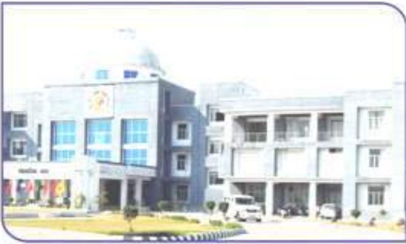
ADMINISTRATIVE BUILDING BUAT, BANDA
